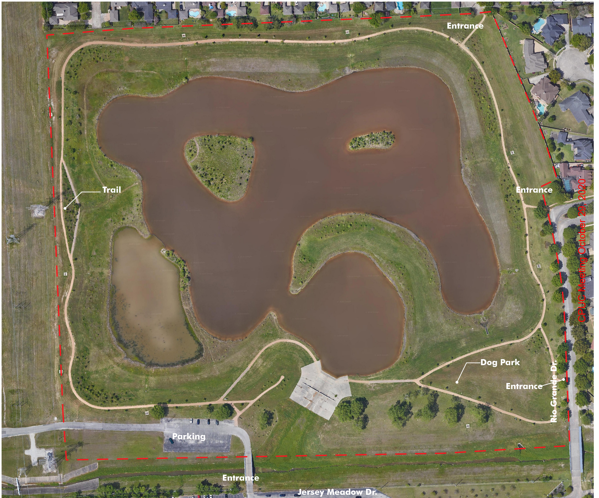
Figure 14. Aerial view of the detention basin.
